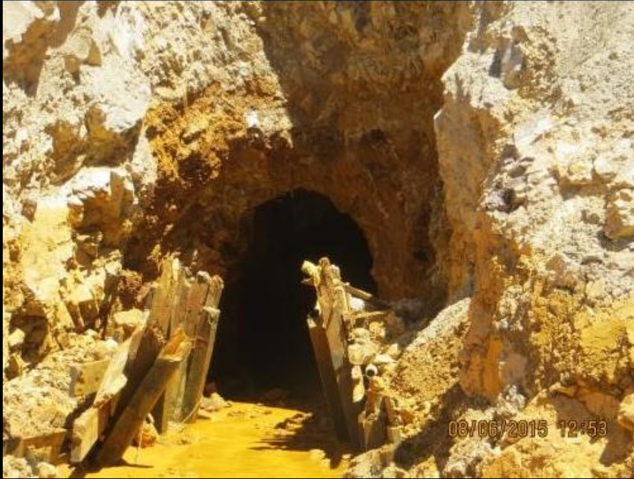
Gold King adit
